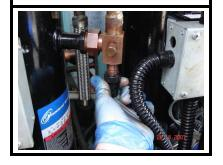
Select compressor, fit service gauges, check pressures.
