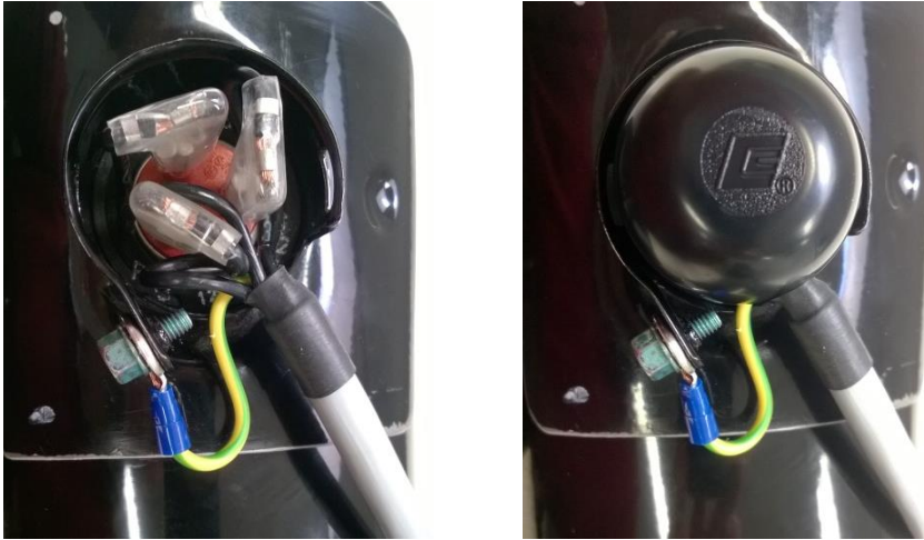
Figure 17: Terminal box and correct electrical installation
