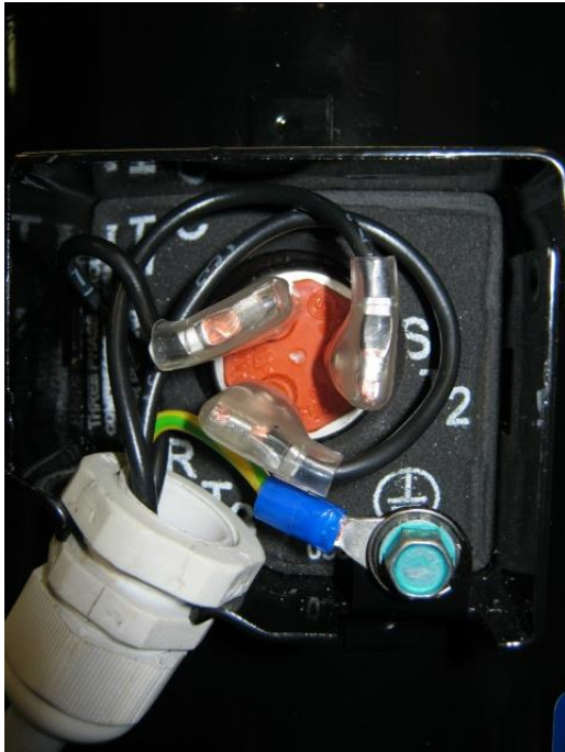
Figure 21: Correct electrical installation with cable glands for IP21 T-box, eg, model ZH04K1P
