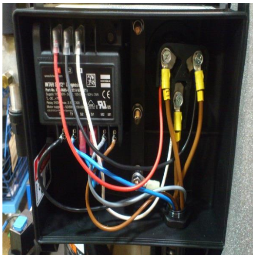
Figure 22: Correct electrical installation with cable glands for IP54 T-box (model ZHI46K1P)
